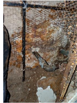
Missing insulation on cold water supply t
