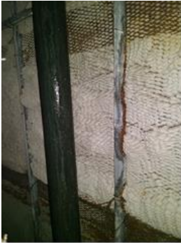
Missing insulation on cold water riser
