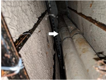
ACM Pipe insulation
