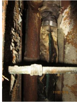
Damaged insulation on cold water riser
